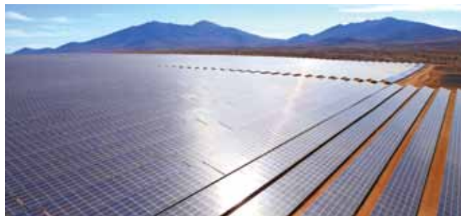
Acciona solar plant in the Atacama Desert
