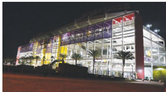
Orlando Stadium using Singbee LED
